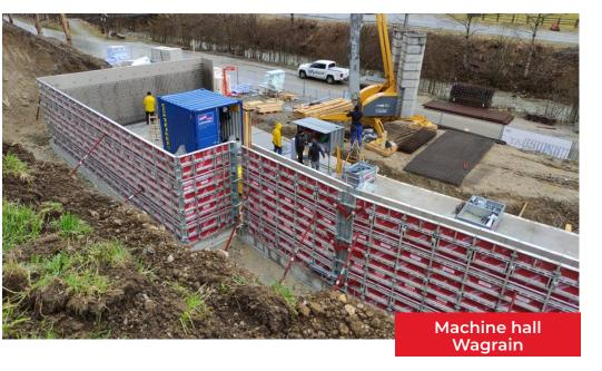
Thanks to perfectly coordinated accessories, such as corners, hinged corners and compensation panels, even complicated floor plans can be implemented quickly.
