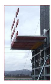
**Concreting platform "L"** for System 2000
