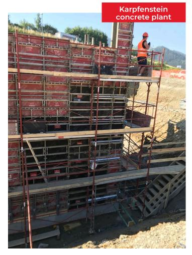
Use over several storeys is no problem at all with System 2000. The variety of panels allows any floor plan to be implemented with ease.
