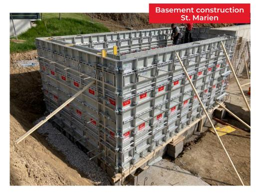
System 2000 with 3m panel height and Alkus solid plastic plywood.
