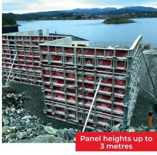
The product range is completed with concreting platforms, brackets, props and brace frames.
