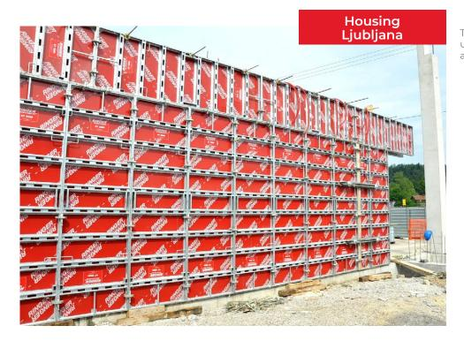
The ST2000 panels can be used vertically or horizontally, as required.
