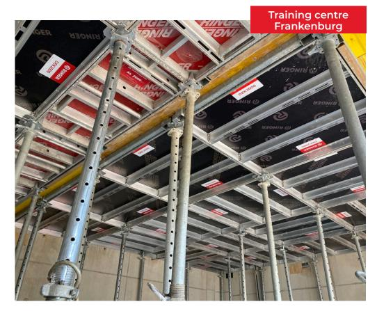
AL2000 in combination with AluDEK is ideal as slab formwork. This minimises infill zones with formwork panels.
